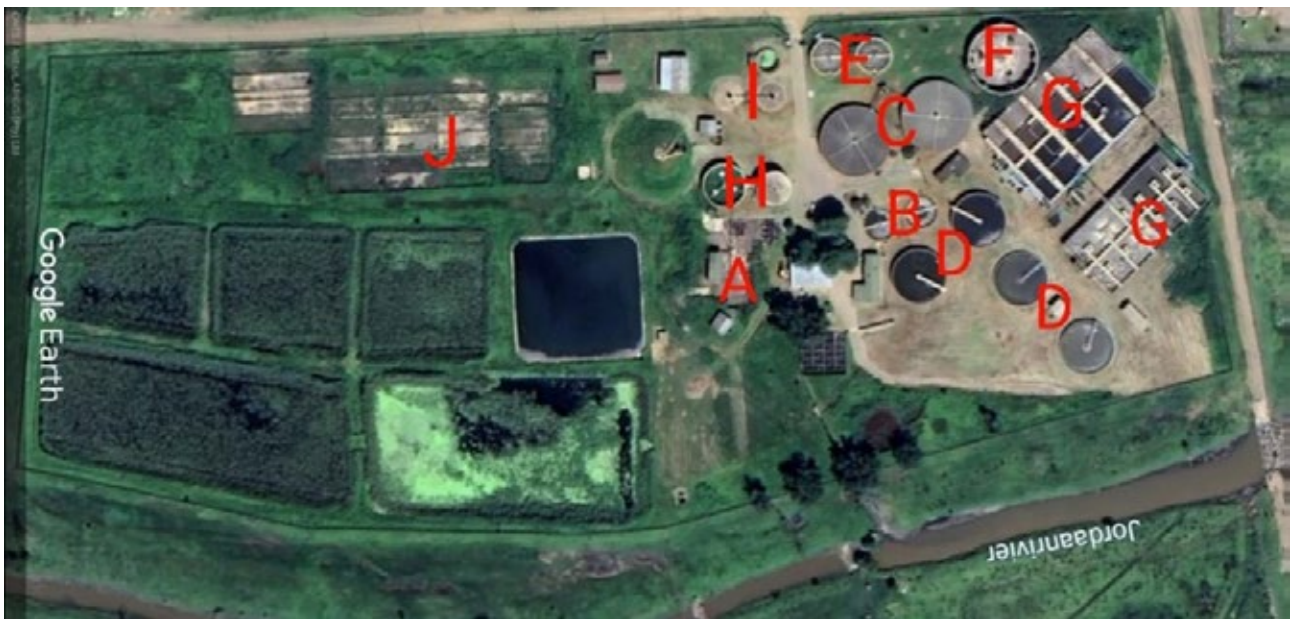
Figure 1.1: Aerial View of Bethlehem WWTP.
