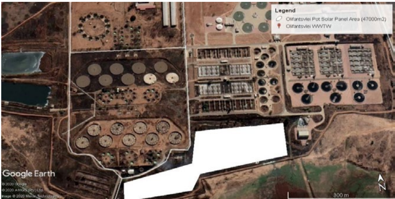
Figure 4.1: Aerial View of Olifantsvlei WWTP.
