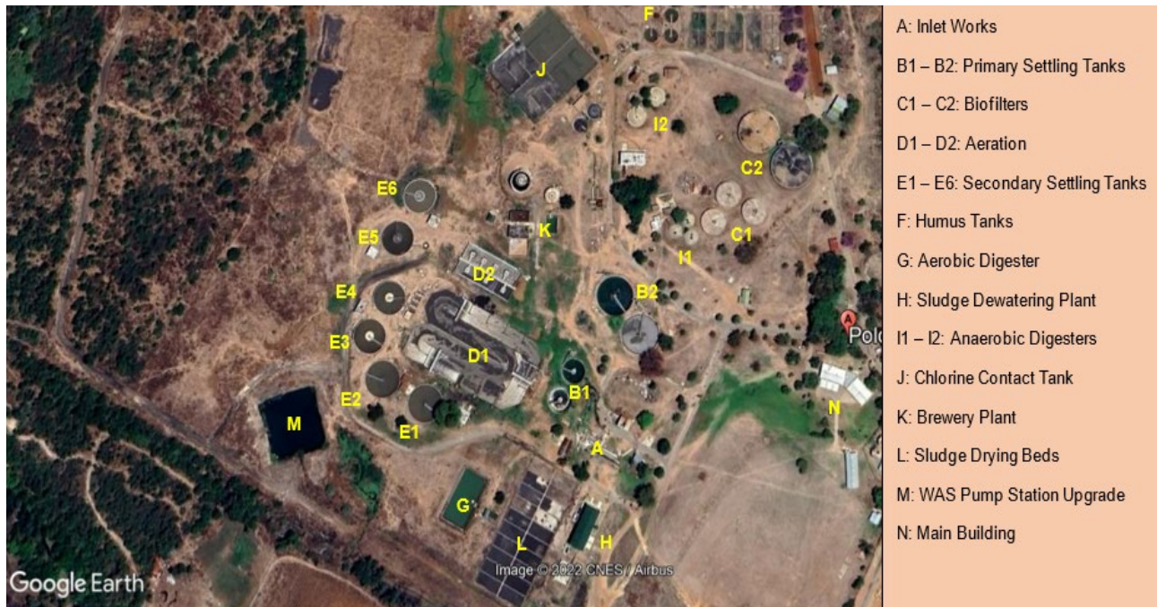
Figure 2.1: Aerial View of Doornkraal Wastewater Treatment Plant.
